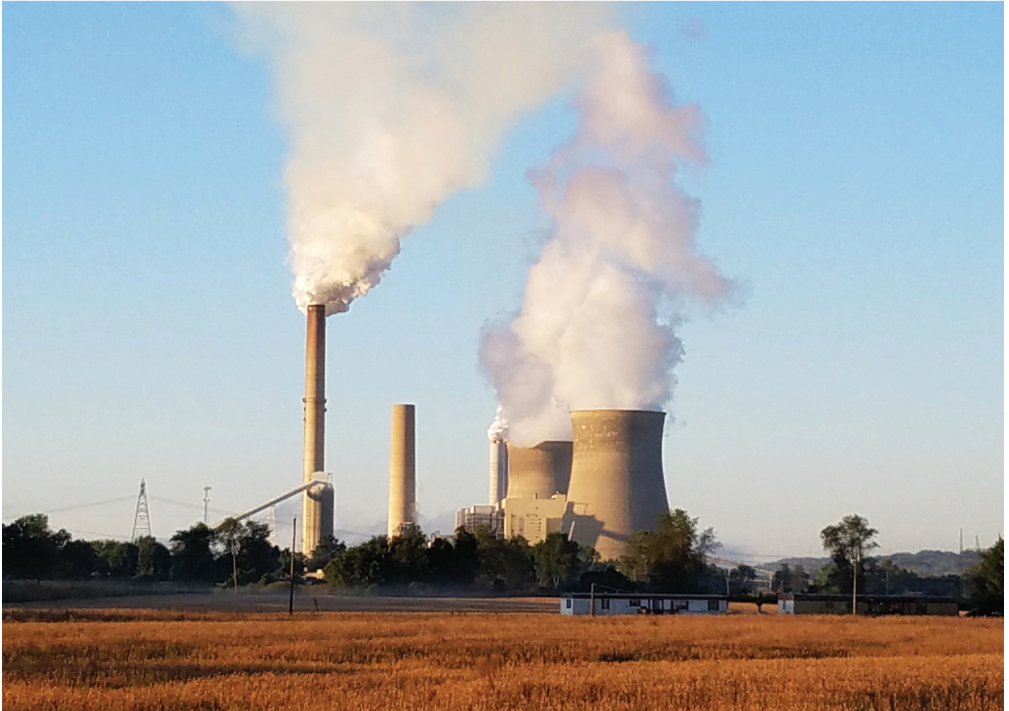
The Gavin Power Plant. Photo copyright Kvaka9/Dreamstime.com
