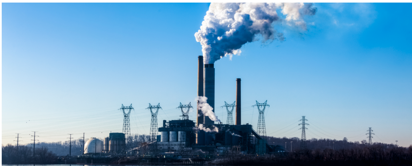
BRUNNER ISLAND COAL PLANT IN PENNSYLVANIA PHOTO: DRNADIG/ISTOCK.COM
